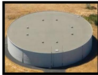
Fig 1.1 Ground water tank
